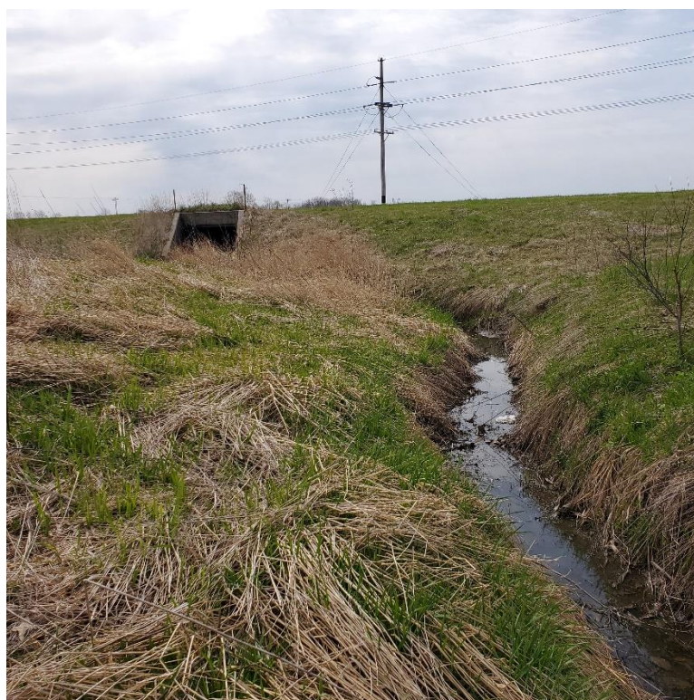
Photo 8: View of tributary running through the site, near the Highway 22.
